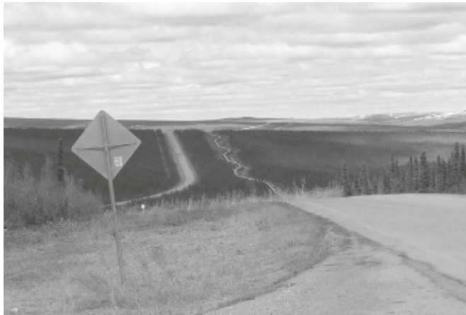
TRANS ALASKA OIL PIPELINE ALONG DALTON HIGHWAY
