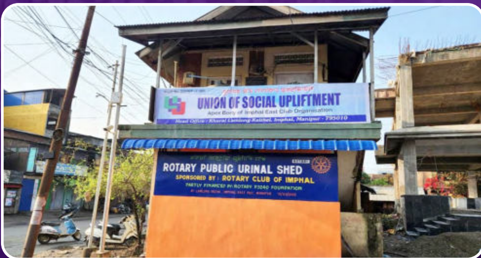
“Rotary Public Urinal Shed” constructed under the District 3240 Foundation at Lamlong Bazar, Imphal East being handed over to the public on “World Rotaract Day”, 13 th March , 2022
