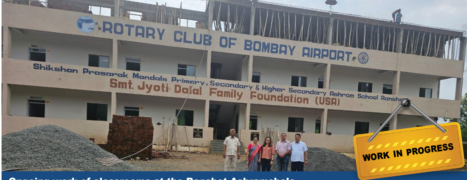
Ongoing work of classrooms at the Ranshet Ashramshala
