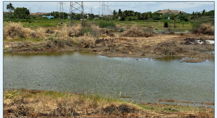
ROTARY CLUB OF MADURAI BLOSSOM WORK COMPLETED AT THATTANUR
