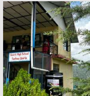
Rain Water Harvesting at GHS Sanhog
