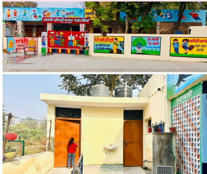
Govt School Renovation
