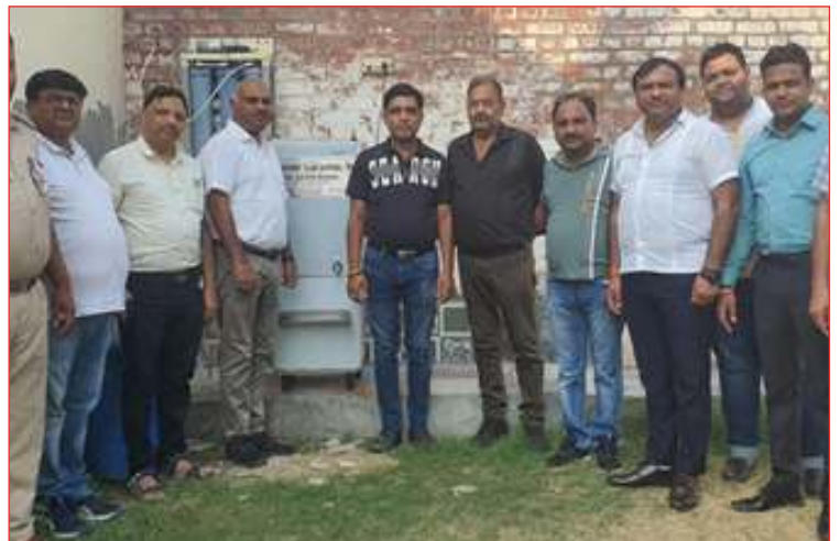
INSTALLATION OF WATER COOLER AT WOMEN CELL IN DISTRICT JAIL
