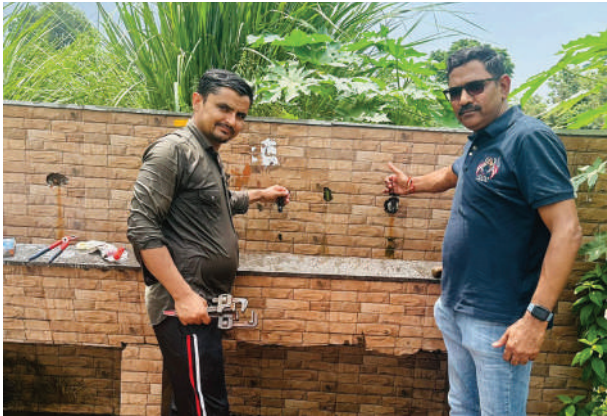
Changing Taps , Pipes and Plumbing requirements at different places
