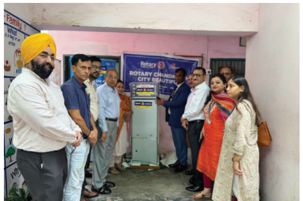
Water Cooler Installed in Govt School, Naya Gaon Mohali
