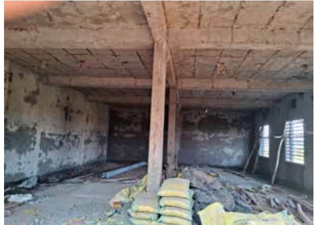
Rotary Bhavan, Morinda at Plastering Phase
